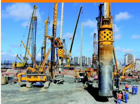
Shaft construction at work.
